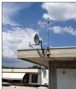
SM with passive reflector for long range connectivity
